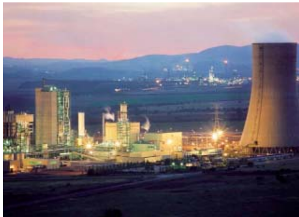
The integrated gasification combined cycle (IGCC) power plant in the Spanish city of Puertollano.
